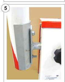
Fasten the M10 nuts onto the bolts and tighten. Fit the end cap to the boom pole.
